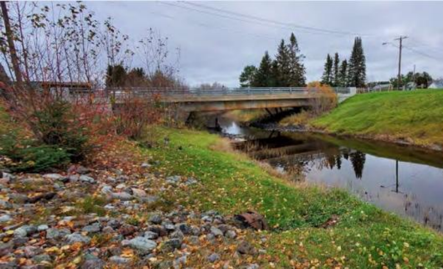
Figure 86: O'Brien Street Bridge - Good Condition (80)
