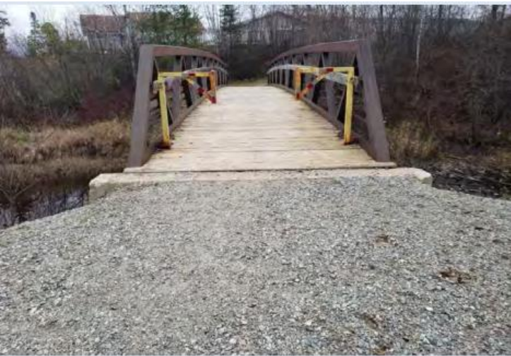
Figure 87: Reid Street Foot Bridge - Fair Condition (40)
